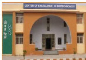
Centre of Excellence in Biotechnology
